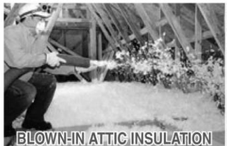
BLOWN-IN ATTIC INSULATION
